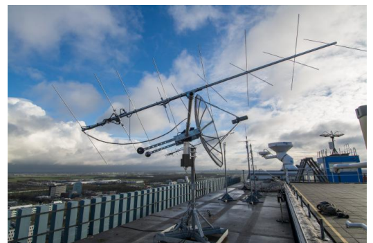
VHF/UHF/S-band 2m Ground Station
